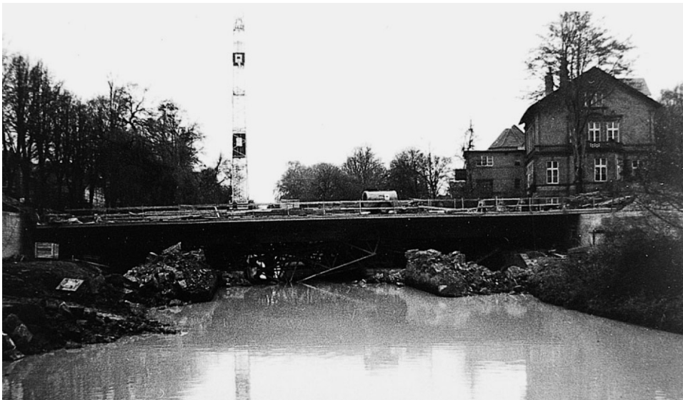
Fig. 11.8 Scaffolding collapses caused by settling of temporary foundations a) Limburg motorway bridge. 1961, Case 11.7 b) bridge in Lüneburg. 1967, Case 11.11
